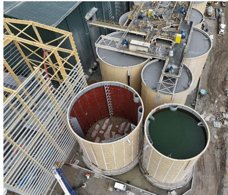
New leach circuit tanks – July 2026
