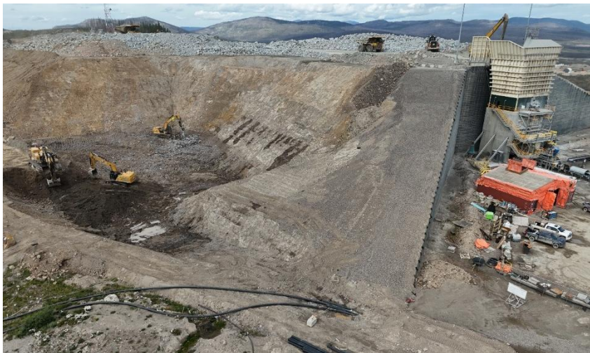
Bulk earthworks for new primary crusher – July 2026
