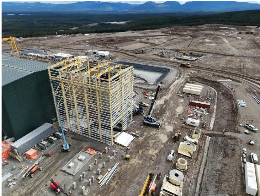
Vertimill building construction – July 2026
