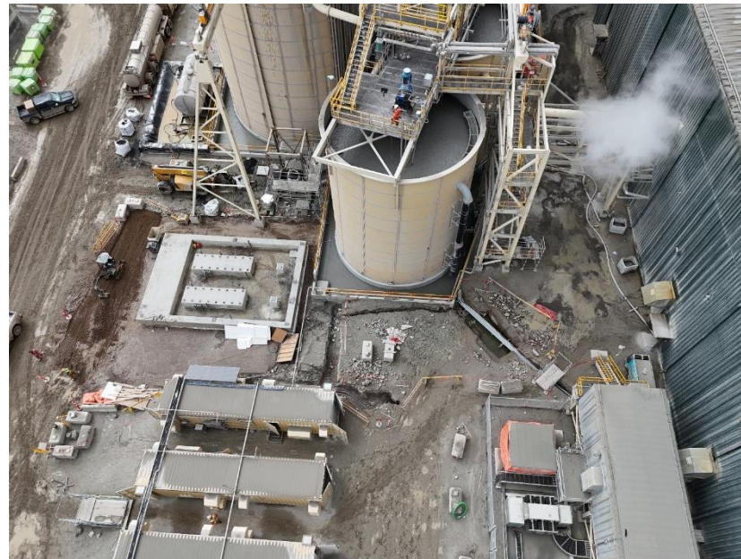
Shear reactor foundations – July 2026
