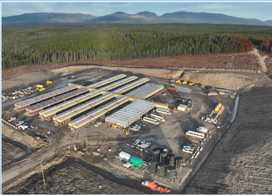
Blackwater's operations camp is complete and has housed operational staff since late Q3 2024.
