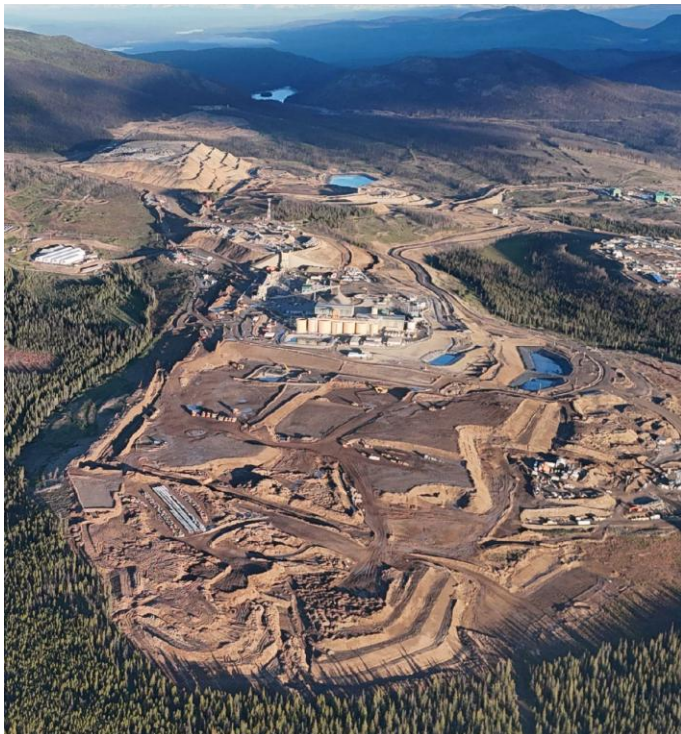
Figure 1 – Bulk earthworks for EP2 processing expansion area – July 2026
