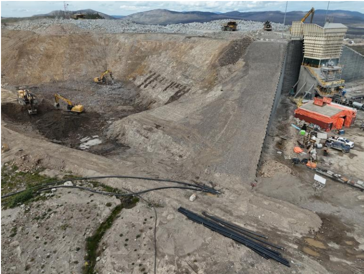
Figure 3 - Bulk earthworks for new primary crusher – July 2026
