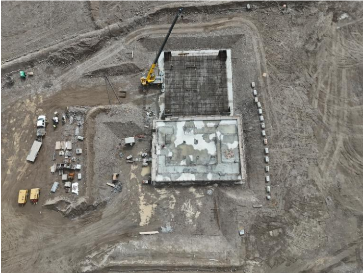
Figure 2 – First concrete pour for EP2 ball mill foundation – July 2026
