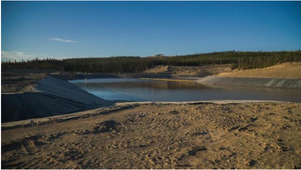
Water management pond
