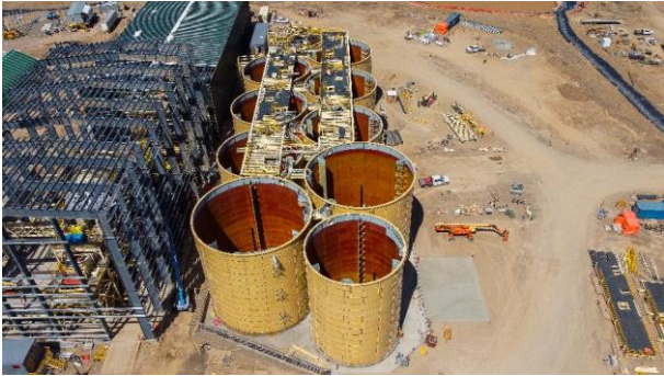
CIL tanks and processing & reagents building
