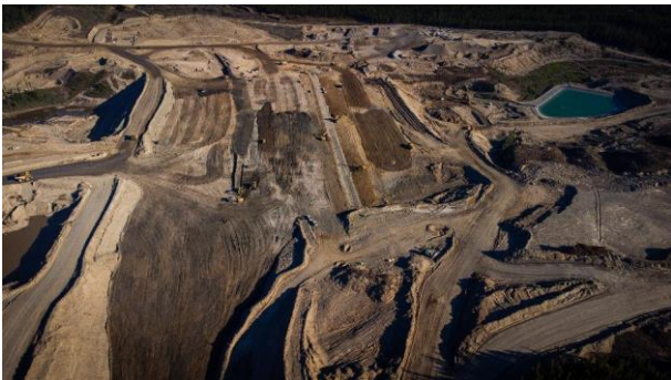
Tailings storage facility
